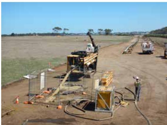
*An HDD rig drilling under a road to avoid the clearing of remnant native roadside vegetation and avoid traffic disruptions during HBWS pipeline construction.*
